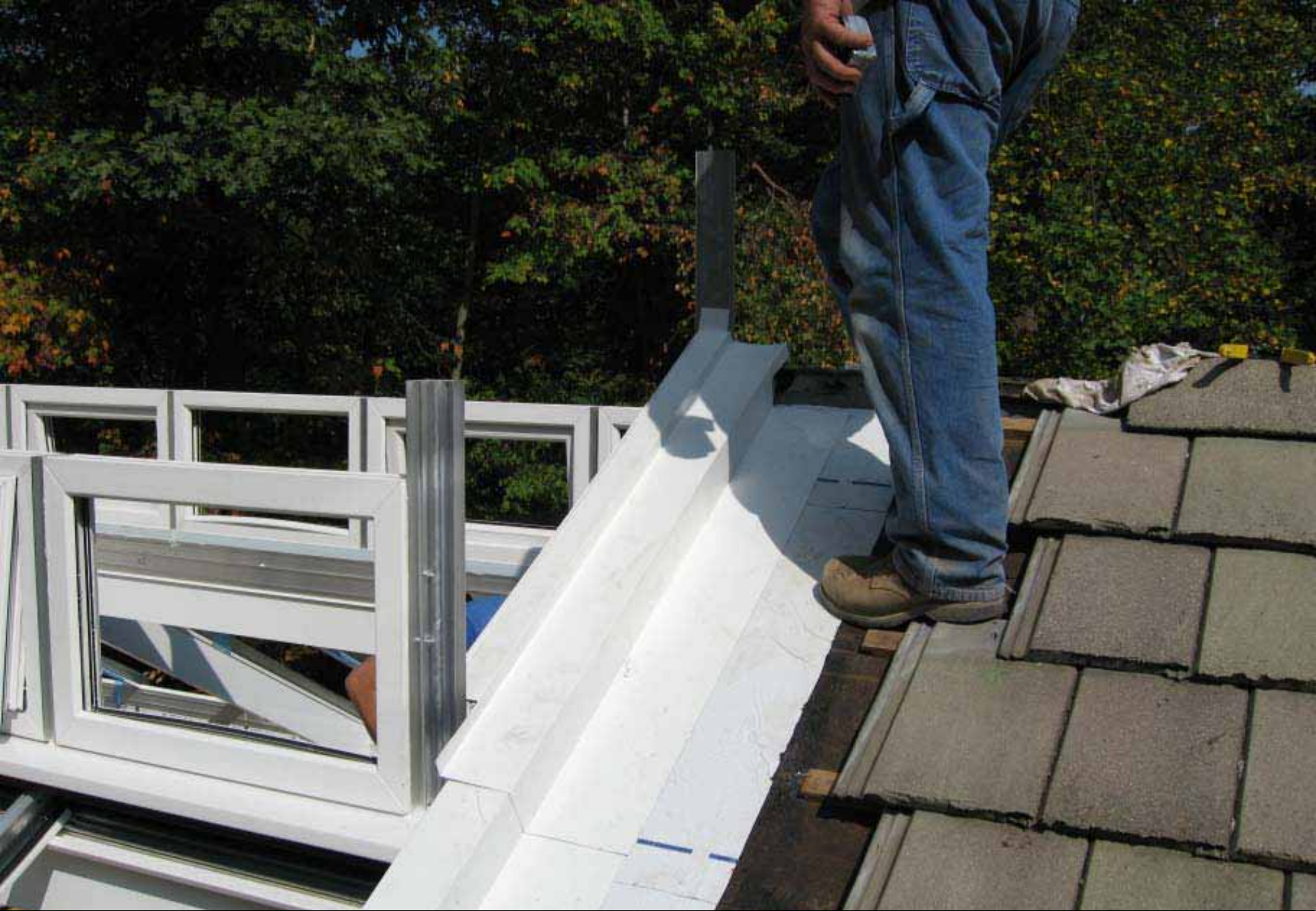
Construction of Lantern Side Fenestration & Flashing
