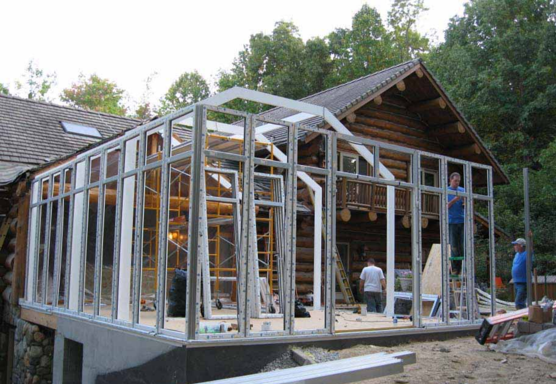
Continuation of Side fenestration Erection
