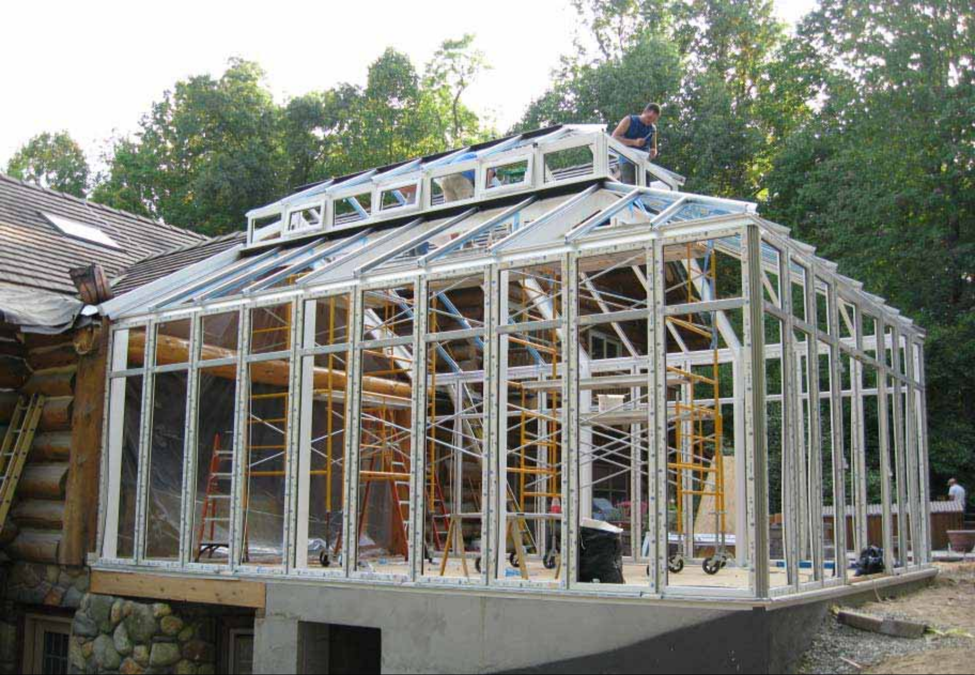
Completion of Lantern Roof
