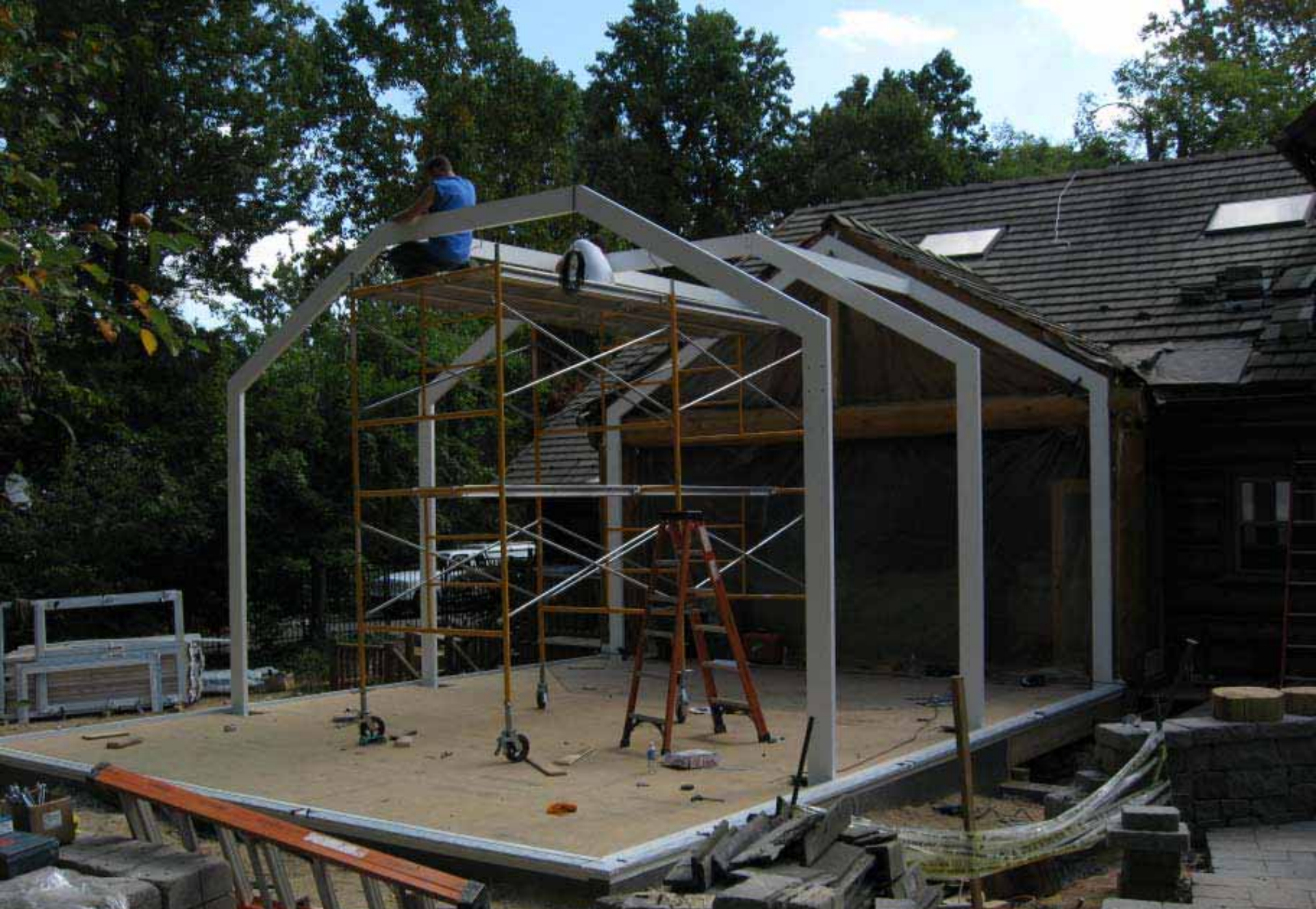
Continuation of Structural Portal Frame Installation
