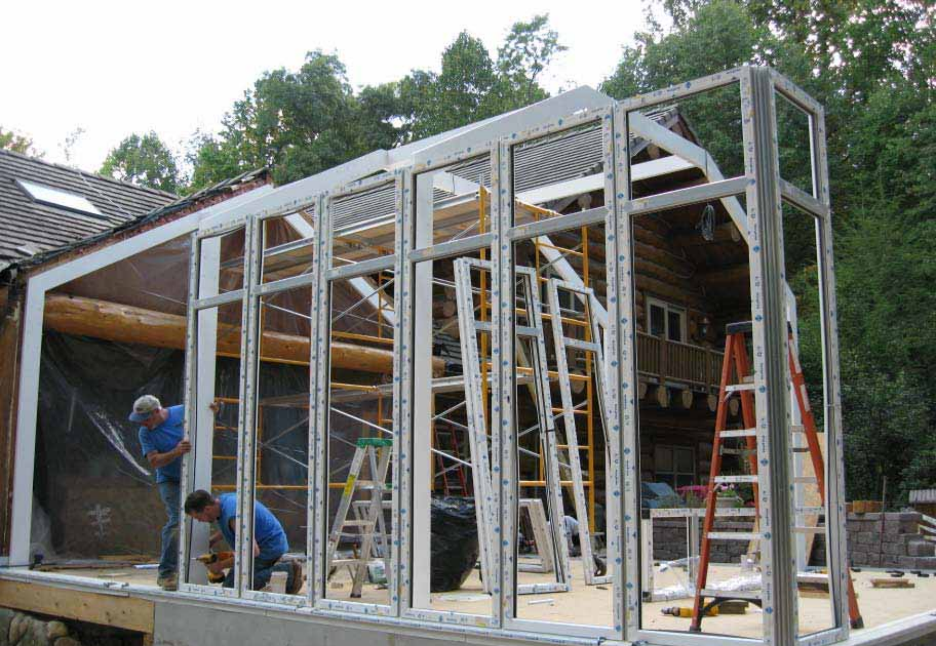
Side Fenestration with Integrated Structural Mullion Supports
