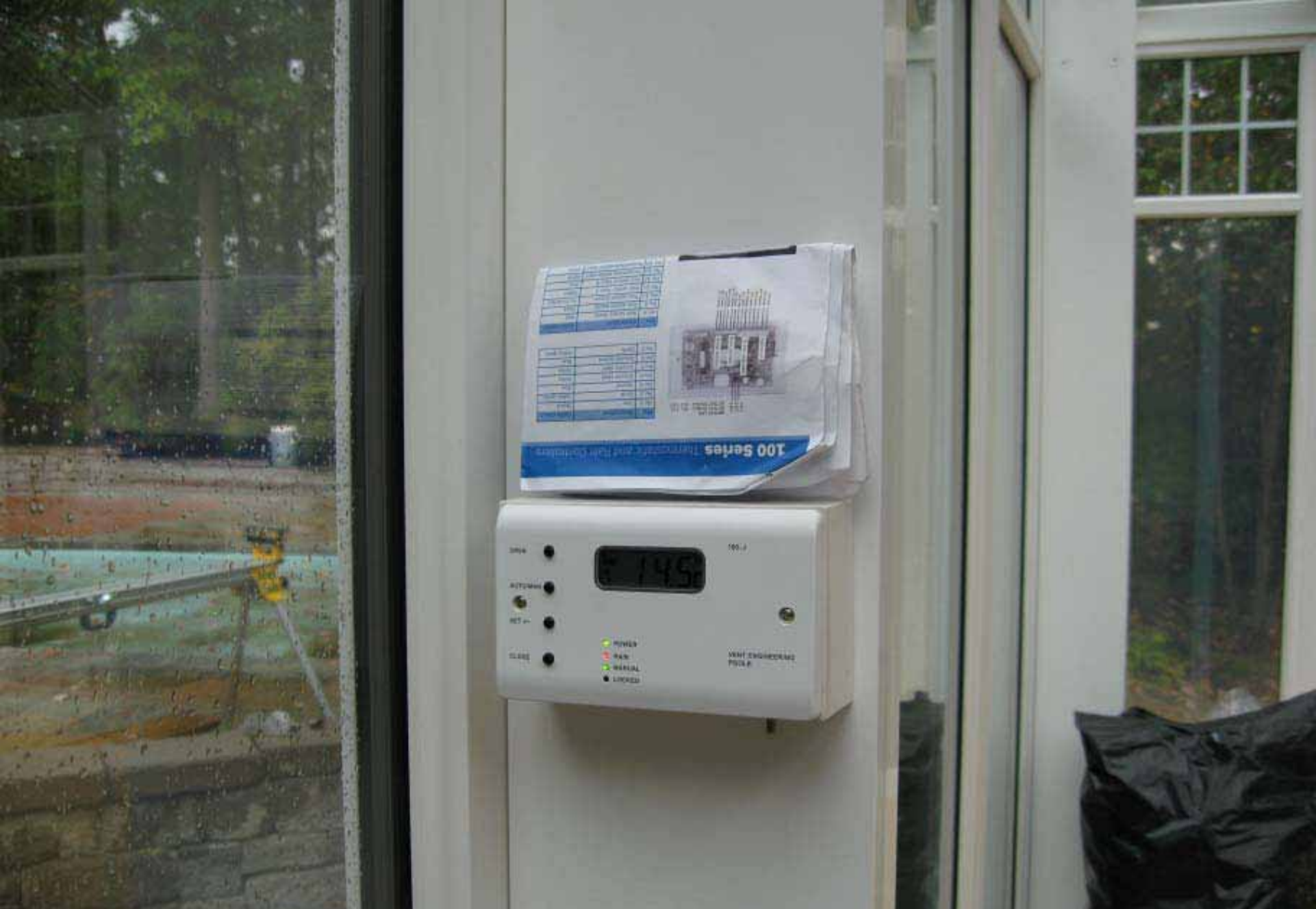
Optional Rain and Temperature Sensor Controller for Motorized Roof Vents
