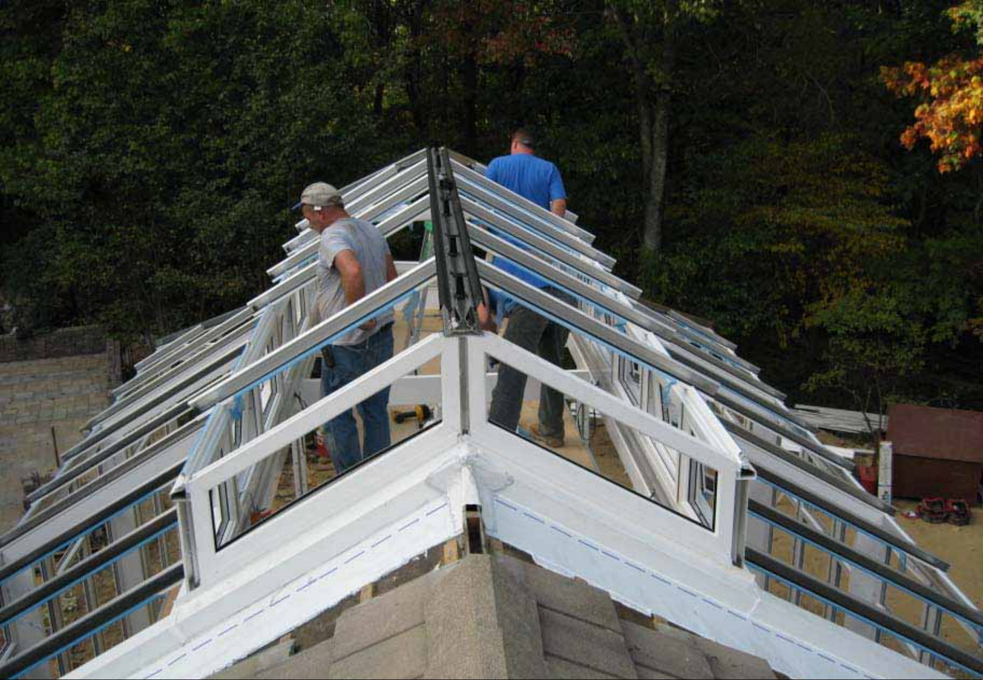
Installation of Lantern Roof Glazing Bars
