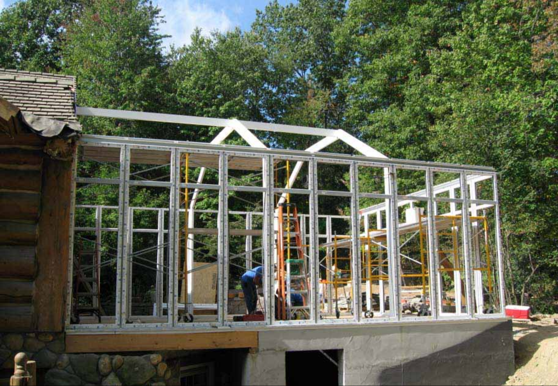
Completion of Side Fenestration
