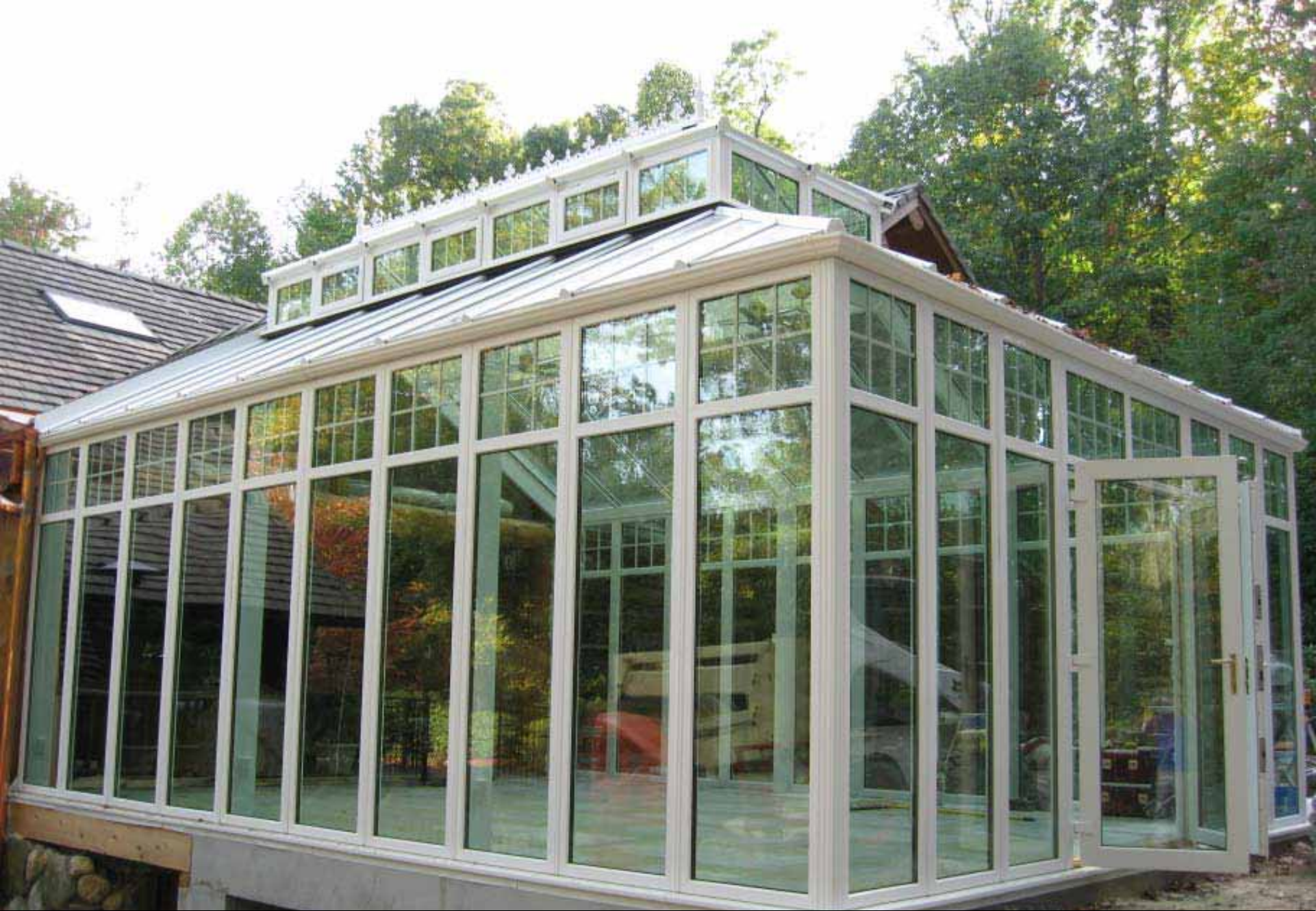
Completed Conservatory Installation
