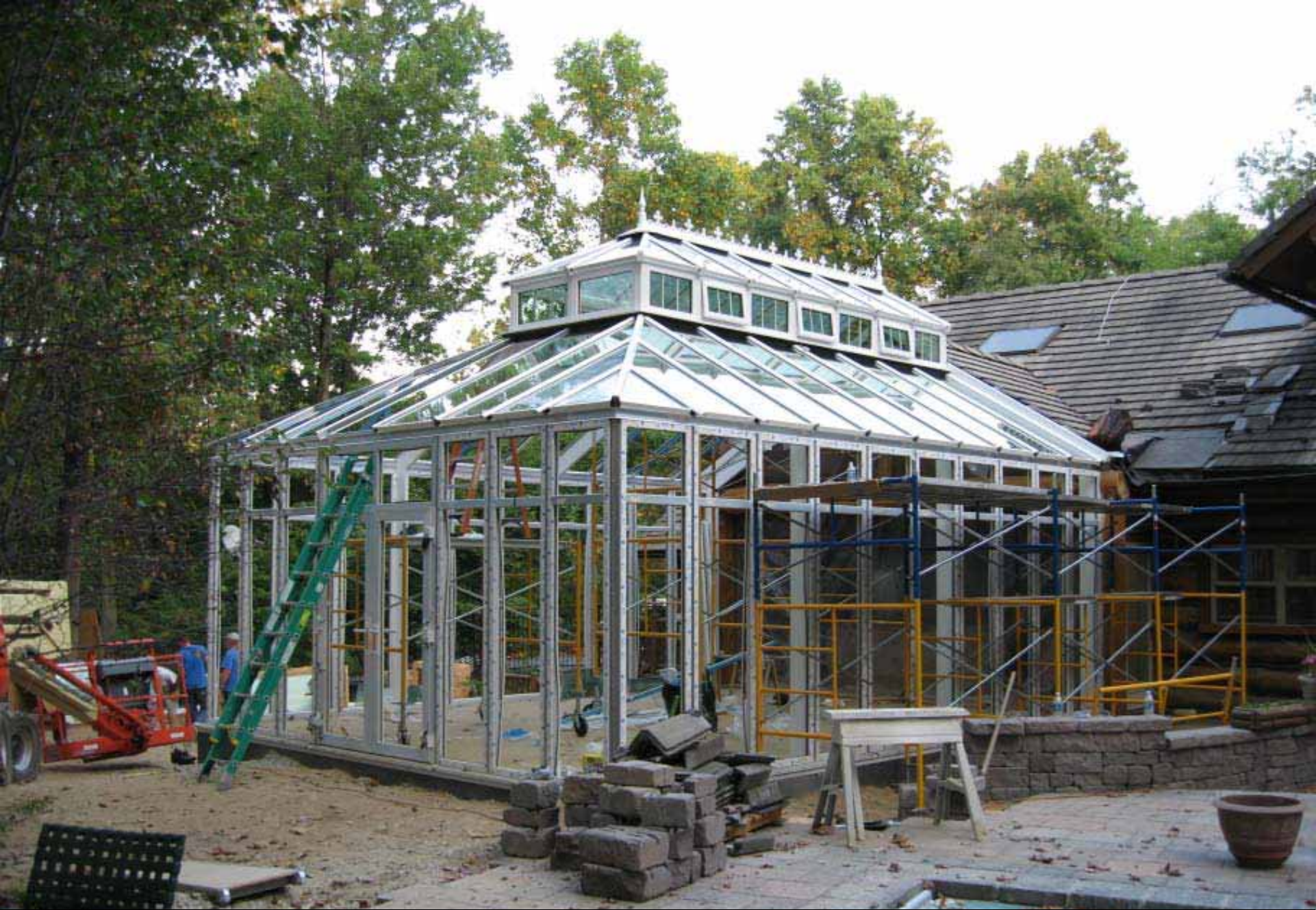
Installation of Main Roof Glazing
