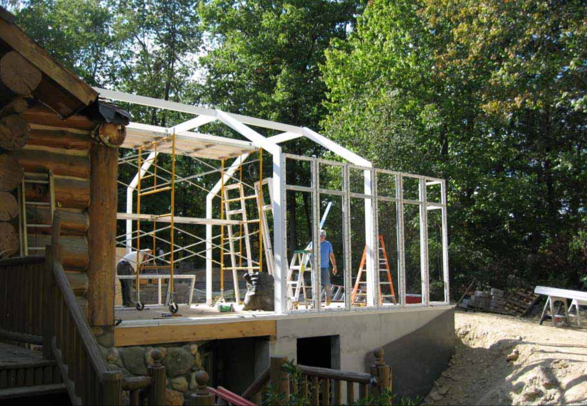
Commencement of Side Fenestration Erection
