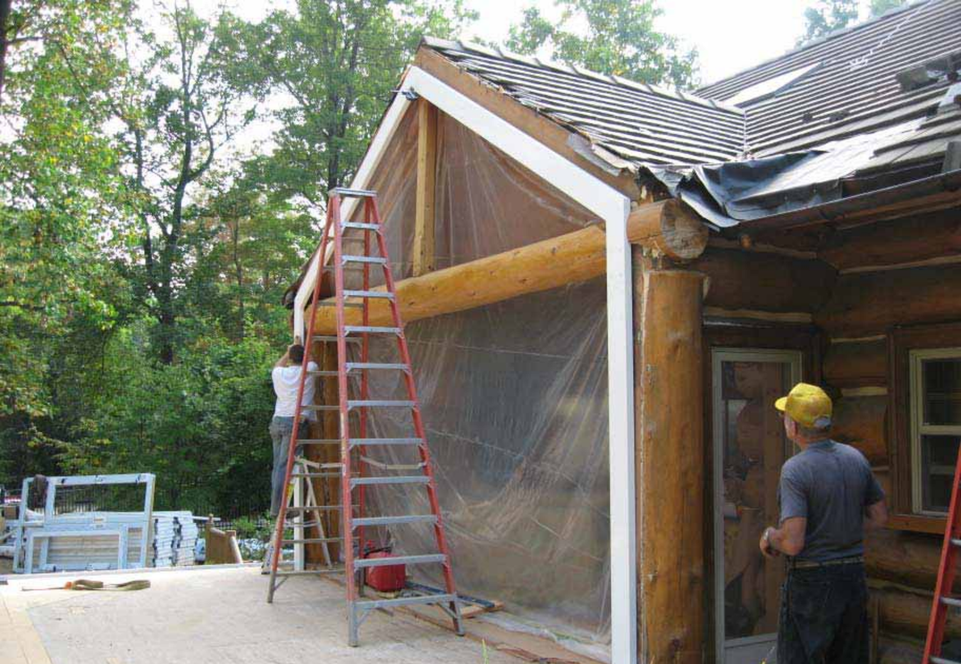
Commencement of Structural Portal Frame Installation
