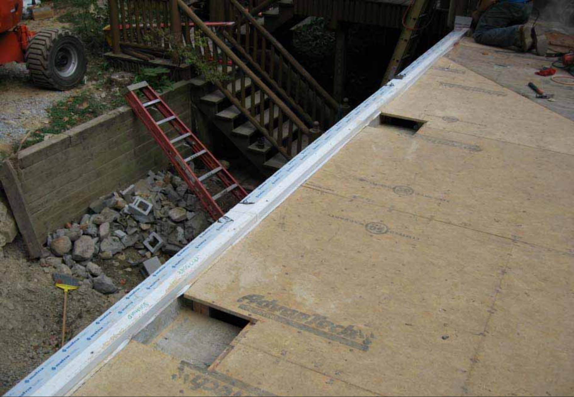
Sill in position + Concrete Piers to support Portal Frame legs
