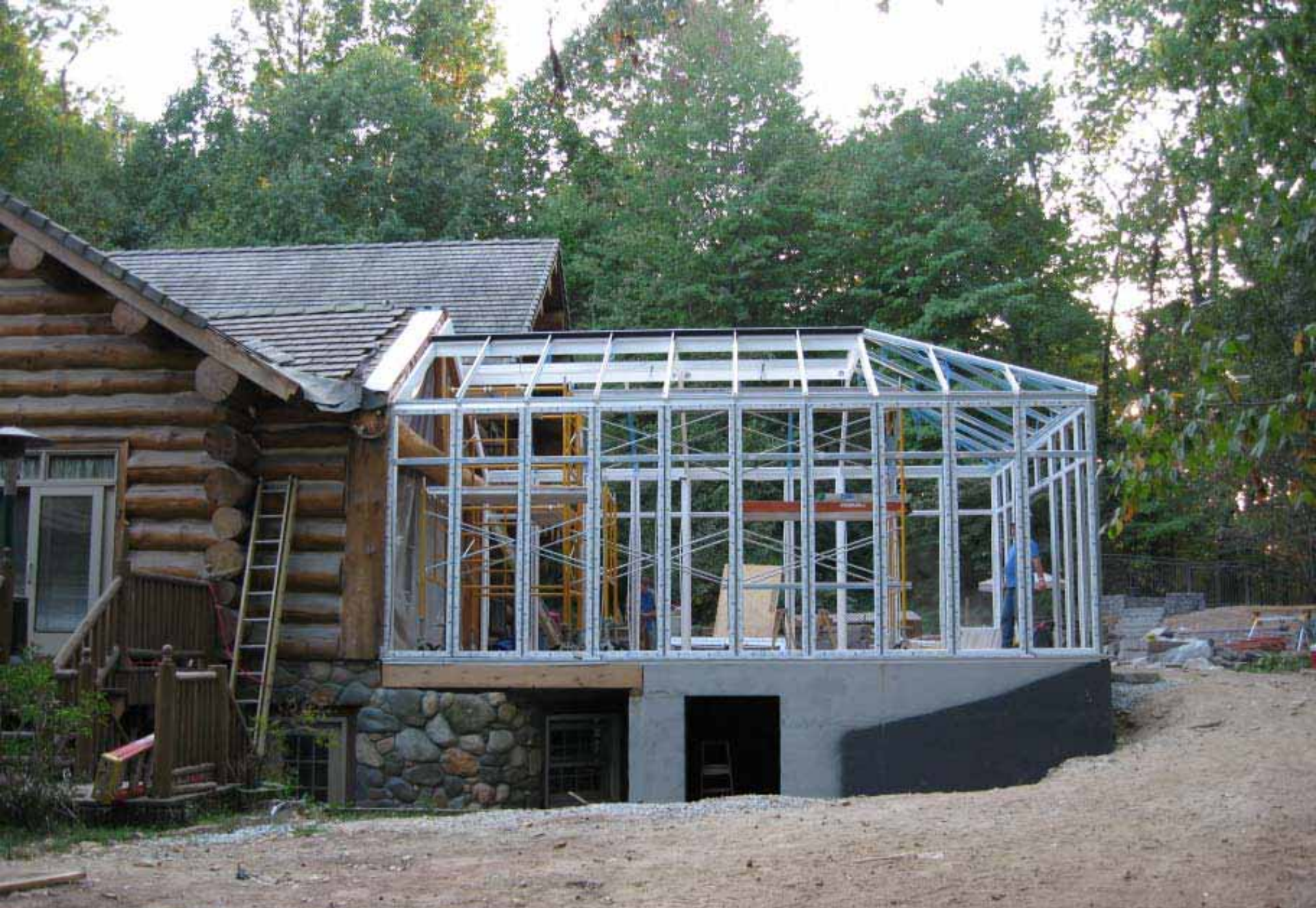
Completion of Lower Roof Glazing Bars
