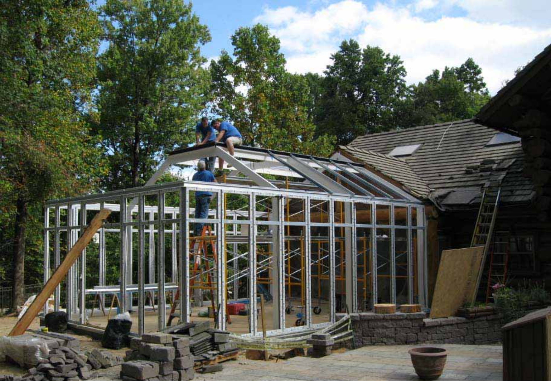
Construction of Lantern Roof and Installation of Lower Roof Glazing Bars
