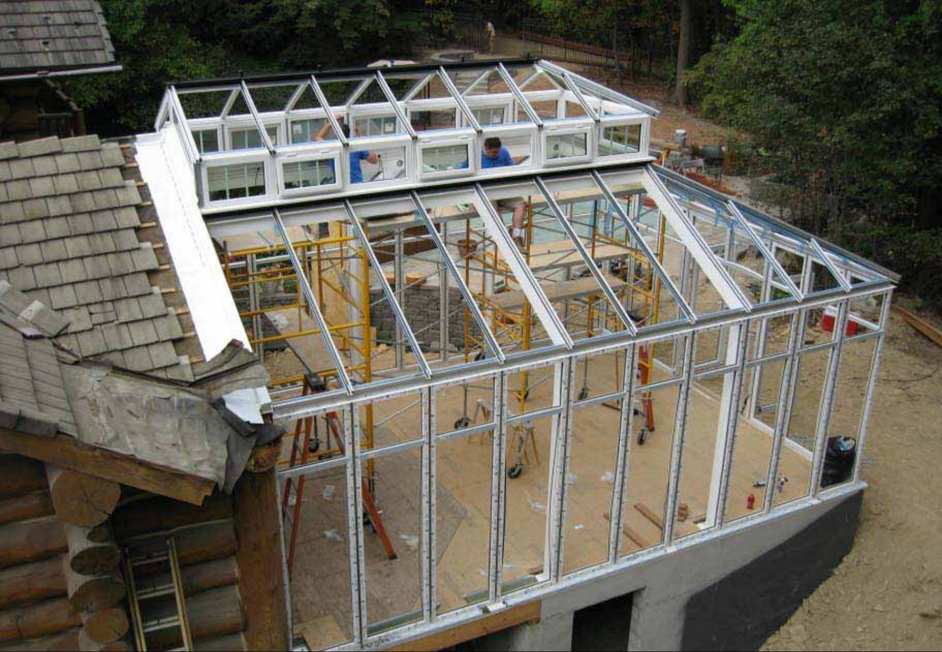
Commencement of Glazing in Lantern Roof
