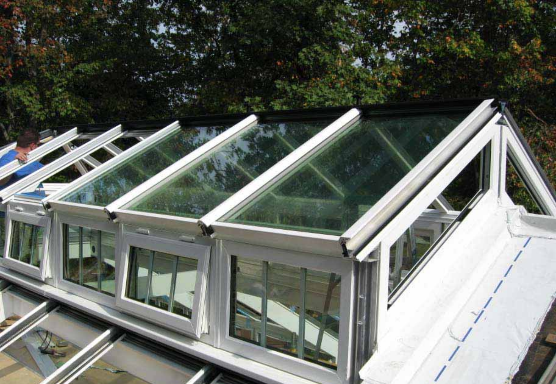
Installation of Glazing in Lantern Roof
