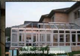
construction in progress
